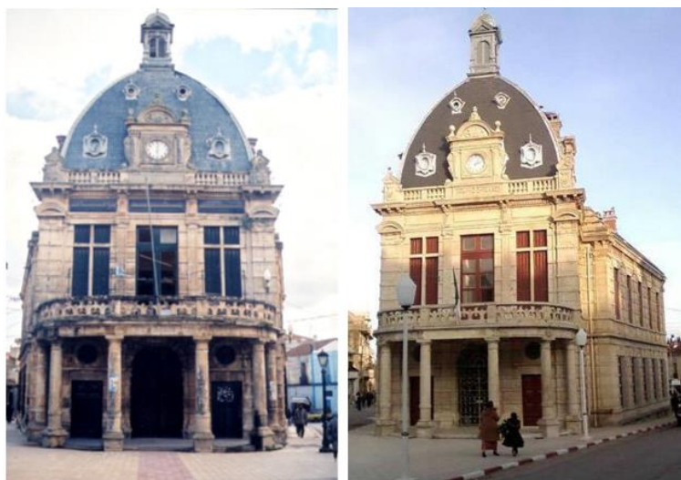
Fig. 2. City Hall before and after rehabilitation
