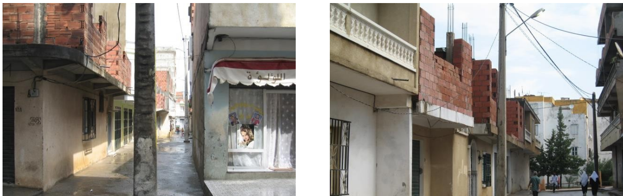
Figure 9. Unsafe proximity of extended balconies to electrical pylons, causing safety hazards, reduced visibility, and visual degradation of façades in « Camp Chevalier » district (Jijel city).
