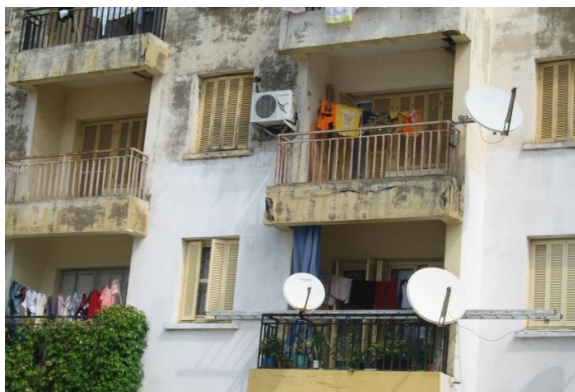
Figure 7. A façade in a deplorable condition due to poor-quality materials and substandard workmanship in Ayouf district (Jijel city).
