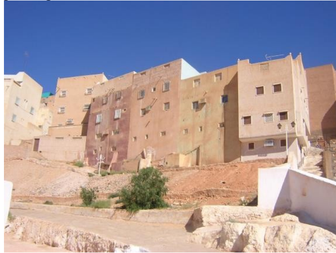
Figure 27. Building façades with small openings in El atteuf Ksar, Ghardaia.
