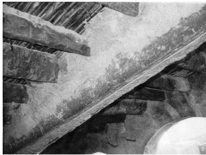
Figure 22. Use of palm brances as insulating materials in roofing in Ghardaïa (Bouchair 2004).
