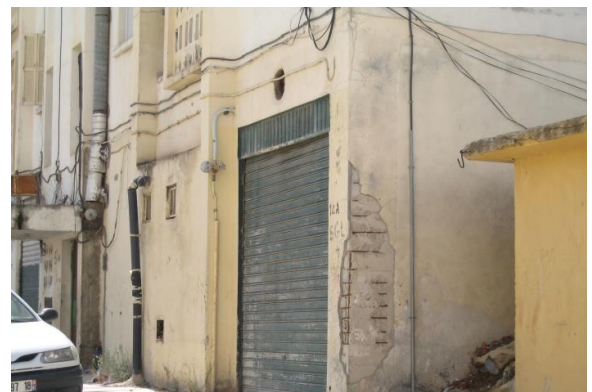
Figure 7. A façade in a deplorable condition due to poor-quality materials and substandard workmanship in Ayouf district (Jijel city).
